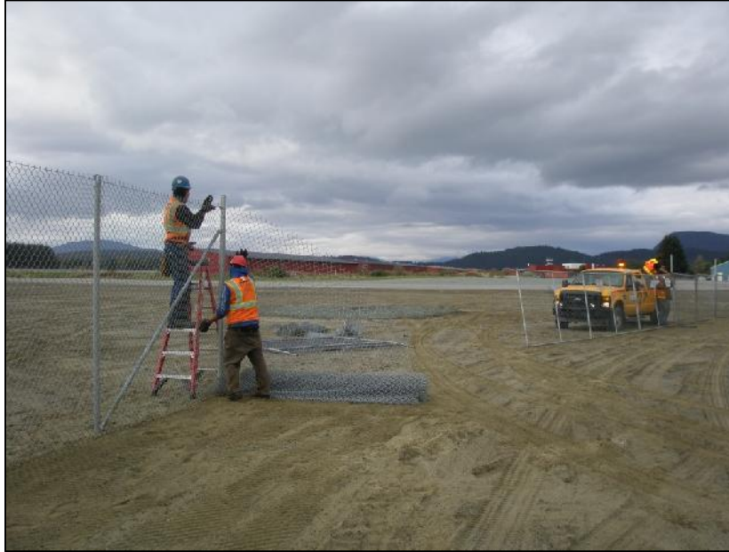
AAA Fence contractors completing installation of south site boundary temporary fence. Juneau Airport maintenance crew was installing portable fencing section.
