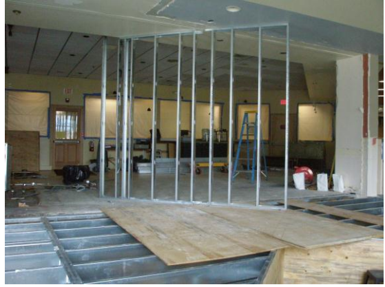
New wall framing for DJ's Tap Room.
