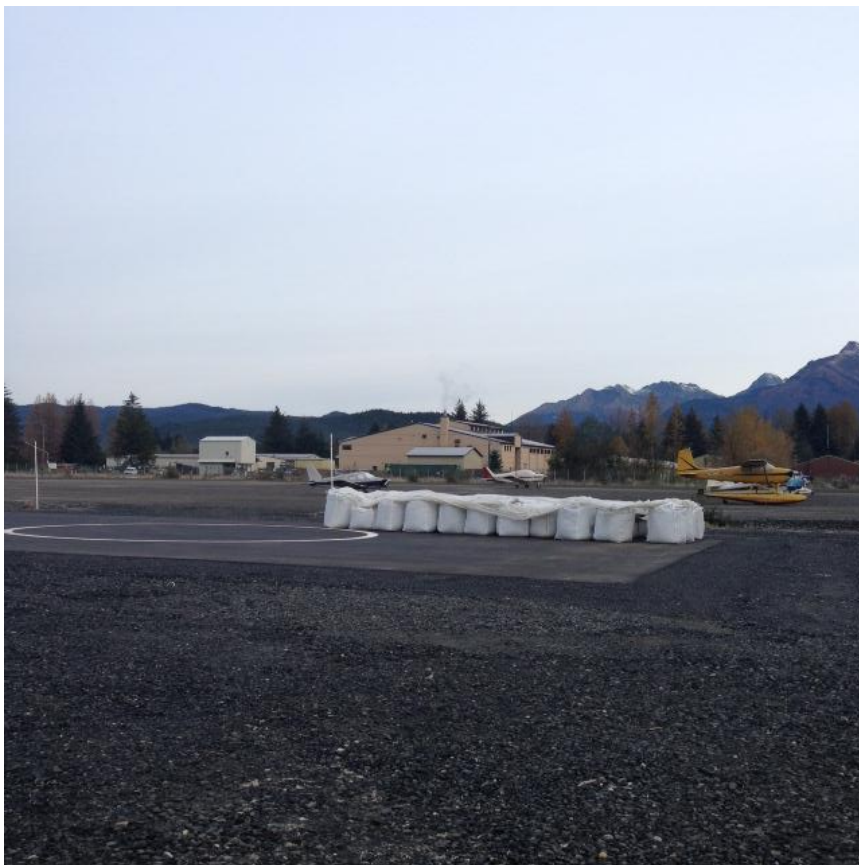
Contaminated Soil Staged on Temporary Helipads
