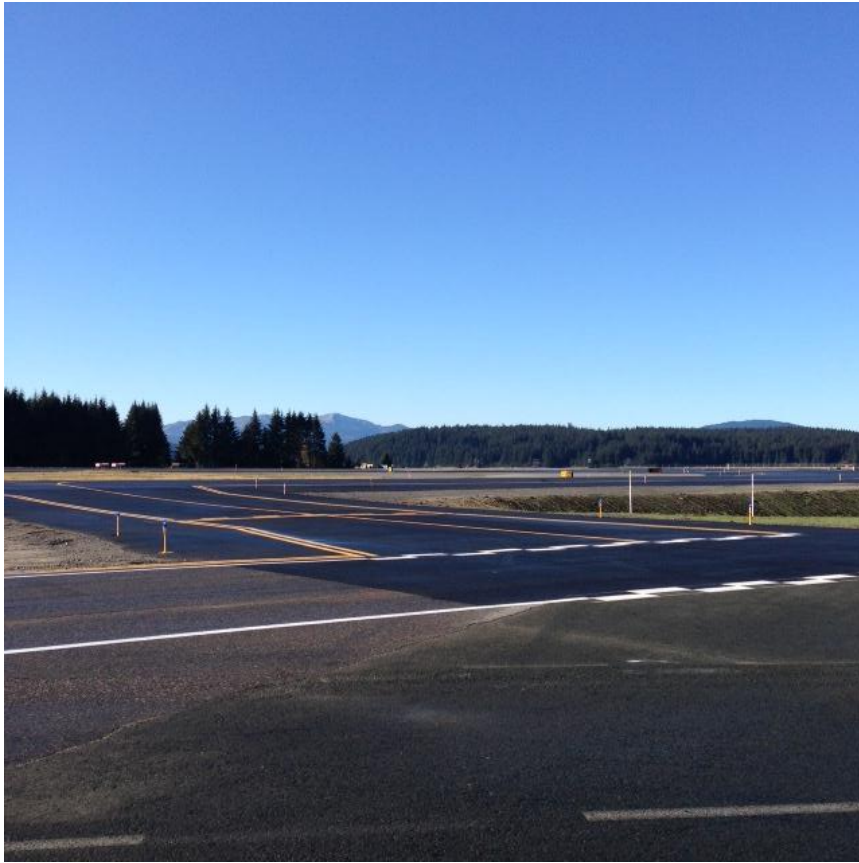
Reconstructed Taxiway B-1
