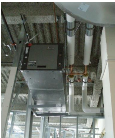
Heat pump #35 set in place.
