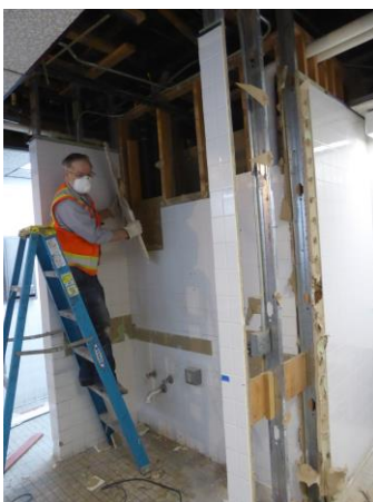
Tile demolition in progress.
