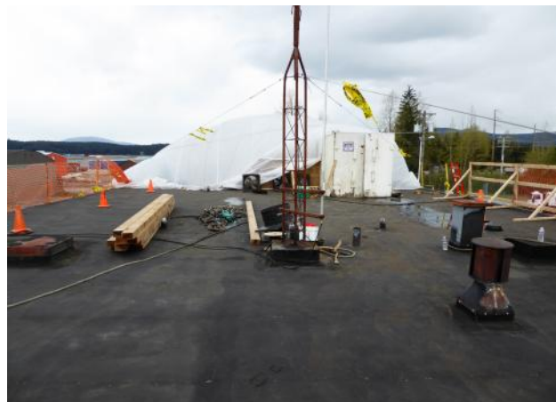
Active work area is enclosed under tent.
