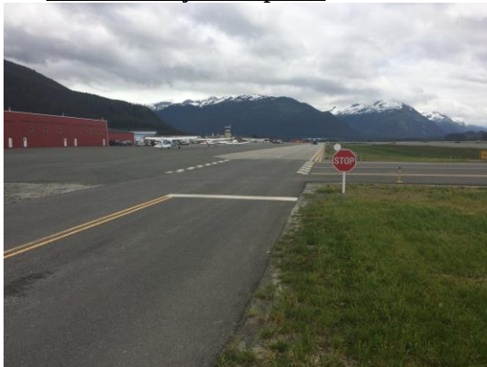
Frangible stop signs on roadways.
