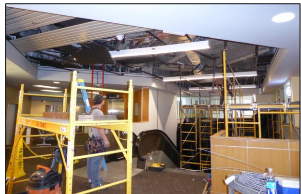
Main stairway lighting upgrades are underway.
