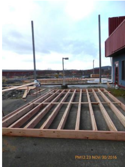
Wall framing at ARFF station constructed on grade; will be placed by crane.
