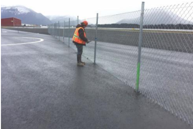
SREB construction area fencing being installed.
