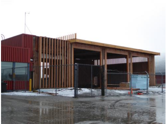
ARFF station, West elevation.
