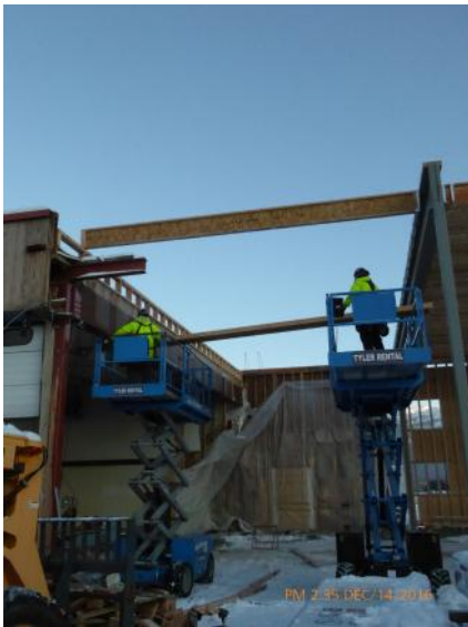
Roof joists being raised at ARFF station.
