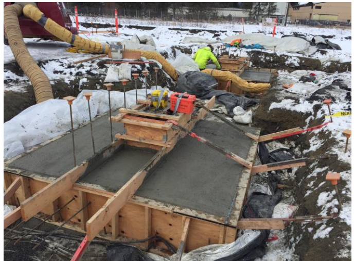
SREB concrete foundations.
