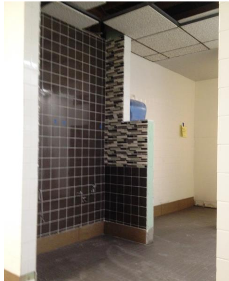
Tile installed in Men's Restroom.
