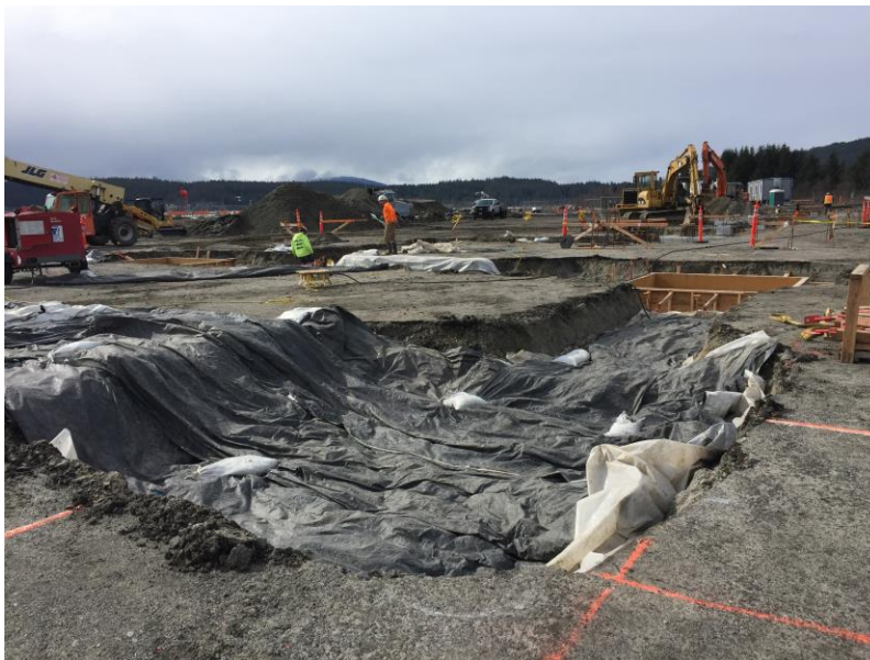
SREB foundation work continues.
