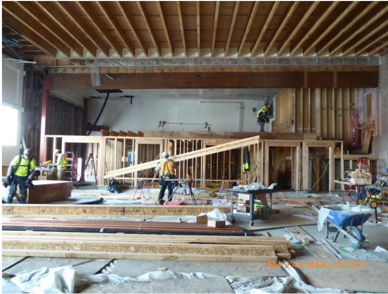
ARFF Station floor mezzanine framing underway.
