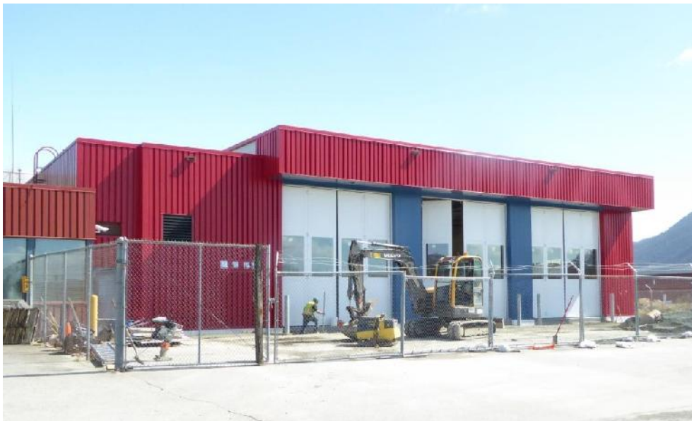
West elevation of ARFF Apparatus Bays.
