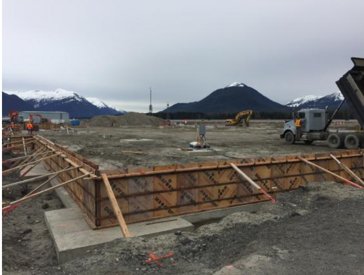
View of SREB construction looking toward Southeast.
