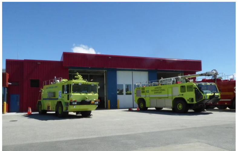
West elevation of ARFF apparatus bays.
