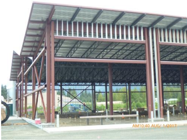
SREB wall framing at southwest bay.
