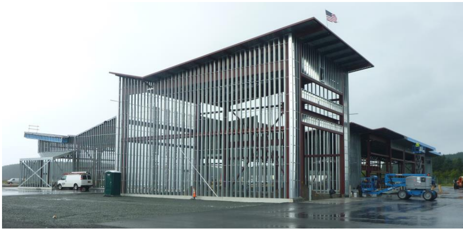
SREB Maintenance Bay
