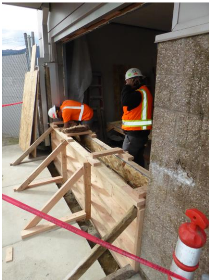
Terminal East Wall Infill
