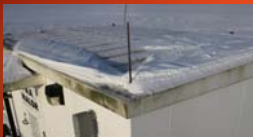
Picture taken from the South East Corner
