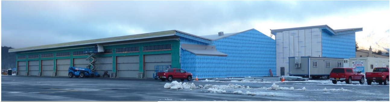
SREB exterior view from southeast corner.
