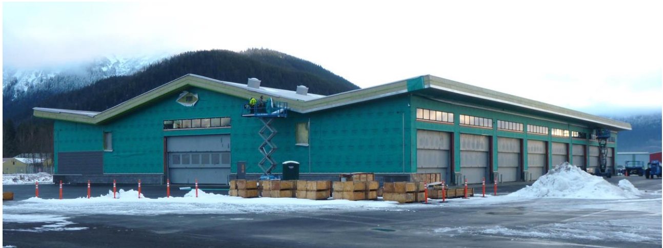
SREB exterior view from southeast corner.
