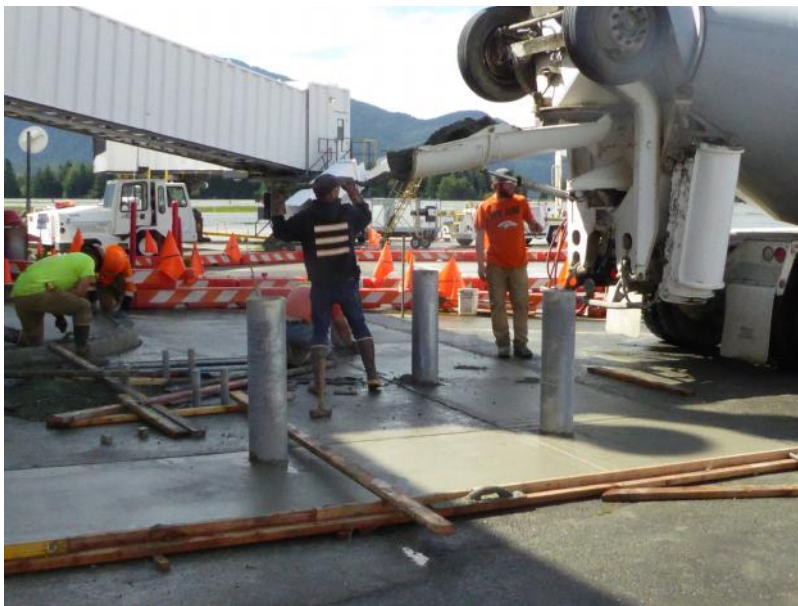
Concrete Placement at Gate 2 Passenger Boarding Bridge.
