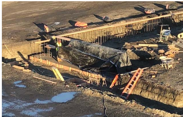
Perimeter excavation and concrete formwork at Sand/Chemical Building
