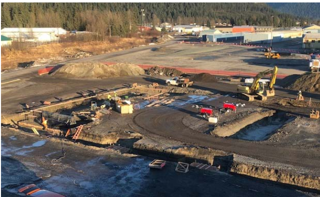
Perimeter excavation and concrete formwork at Sand/Chemical Building
