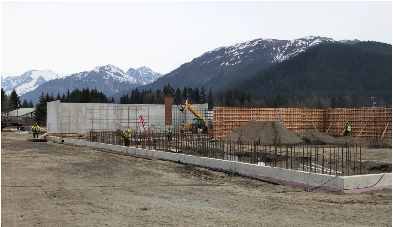
Sand & Chemical Building, looking northeast
