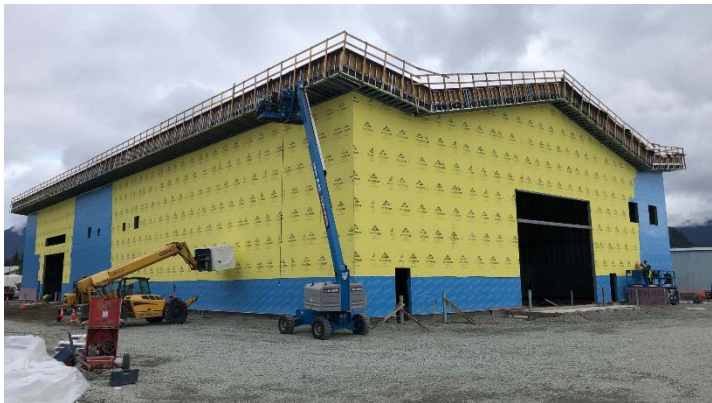
Sand/Chemical Building from SW Corner
