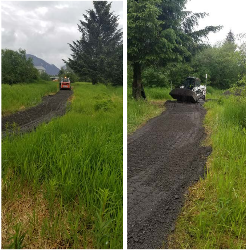
Jordan Creek trail widened/improved
