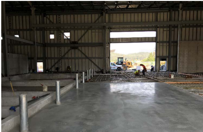
Sand/Chemical Building interior concrete slabs
