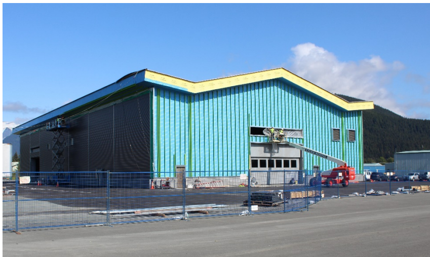
Sand/Chemical Building from SW corner.
