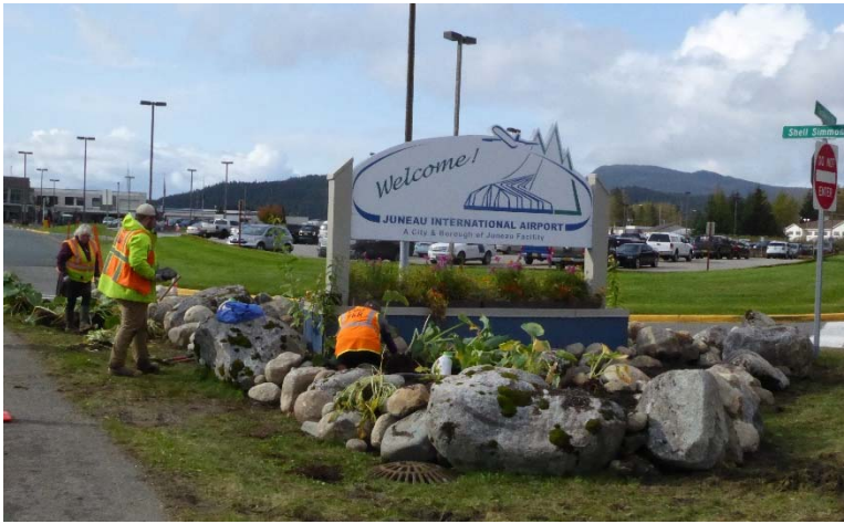
Landscaping transplant at Airport Welcome Sign underway.
