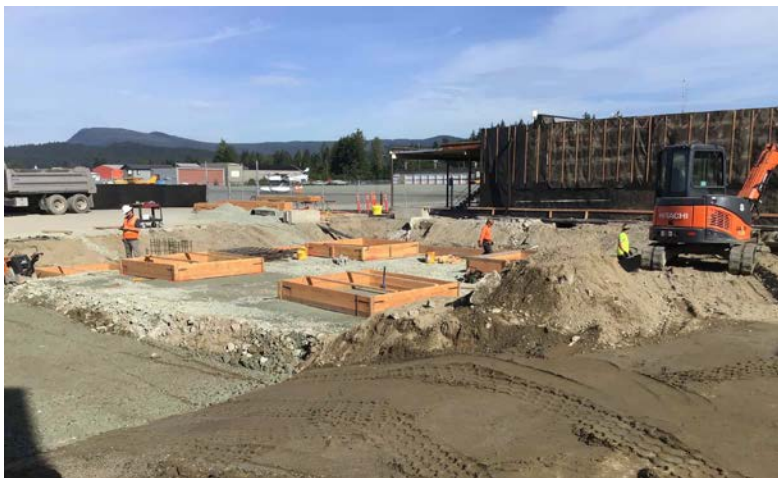
From airside, looking northeasterly into work area.
