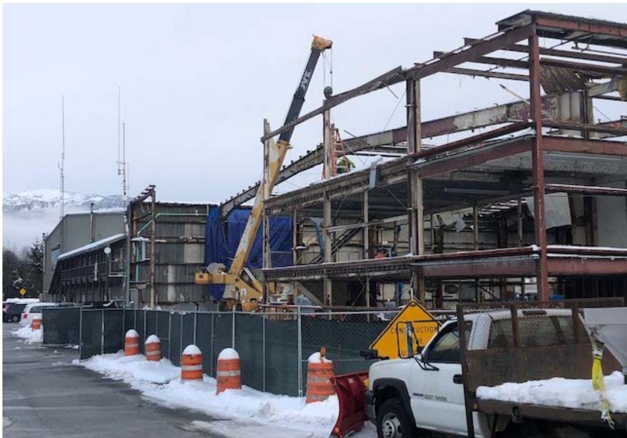
Figure 1-1: Removal of the secondary steel from the roof of the old Sand Shed.
