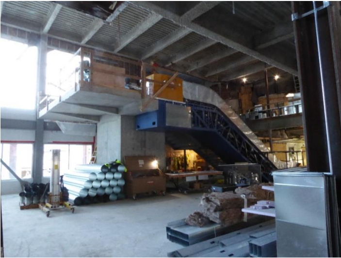
Stair tower with escalator installed.
