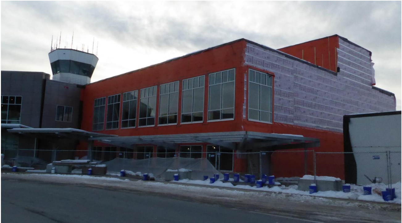
Terminal reconstructed building viewed from Shell Simmons Drive. (Air & water barrier installed over Z-girts with rigid insulation.)
