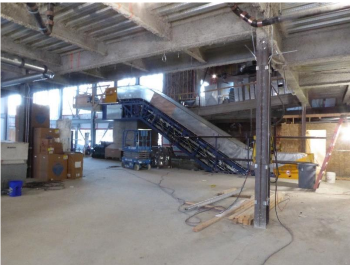
Escalator & ramp viewed from west seating area.
