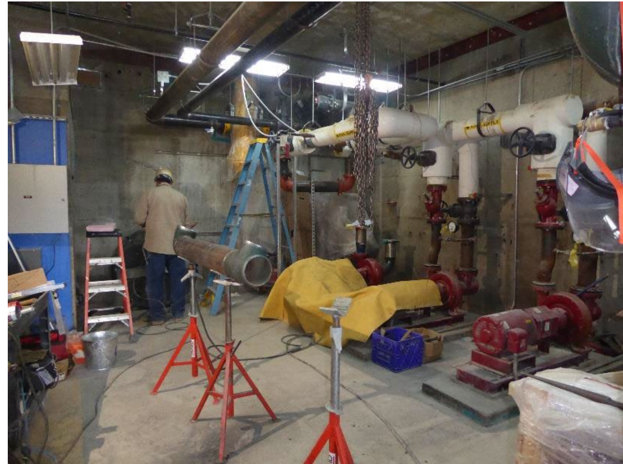
Ground source heat piping install in pump room.
