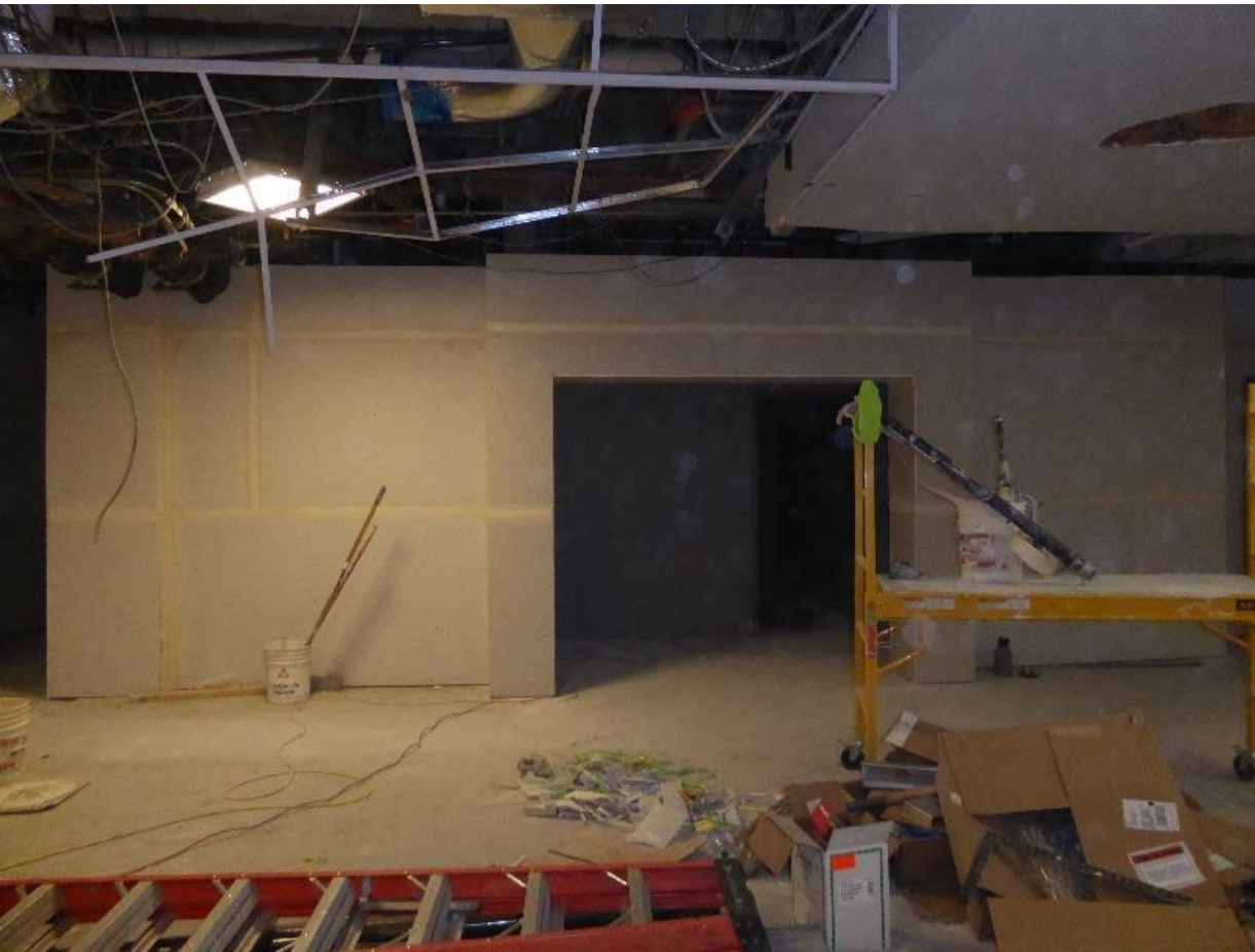
1 st floor toilet room entrance.
