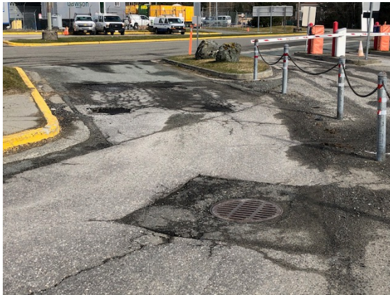
Taxi staging lot entry
