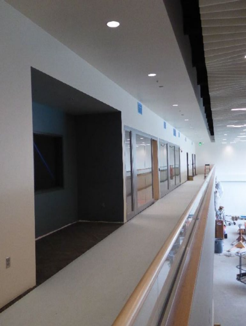
Balcony w/ wood & glass railing installed; admin suites off balcony.
