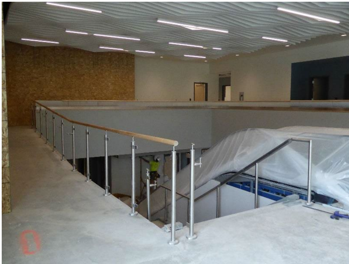
Railing installation in process at stair and ramp.
