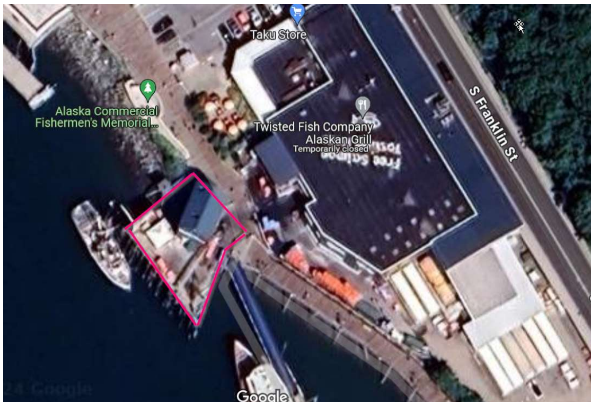
Dock location and current configuration, source Google Earth 2023. Not to scale.
