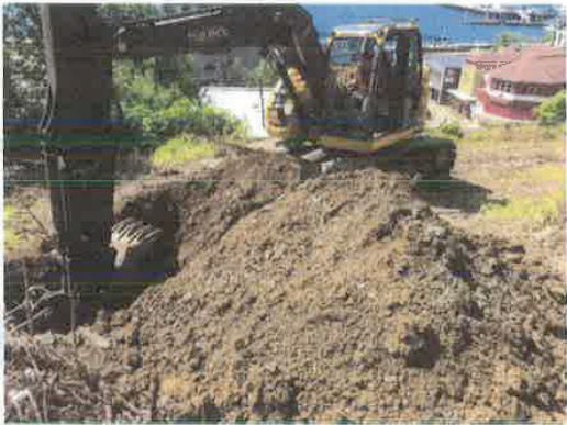
Figure 3: Excavator and in-situ silty sand with gravel
