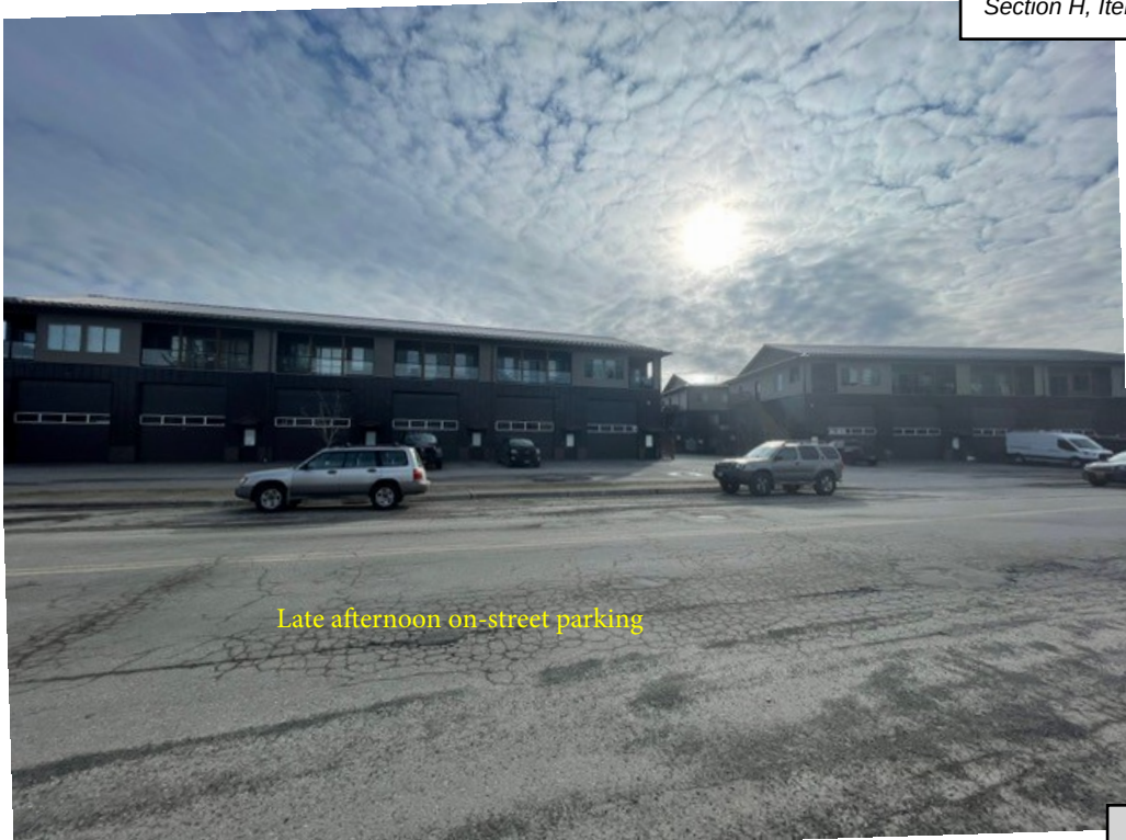
Attachment F - Site Photos
