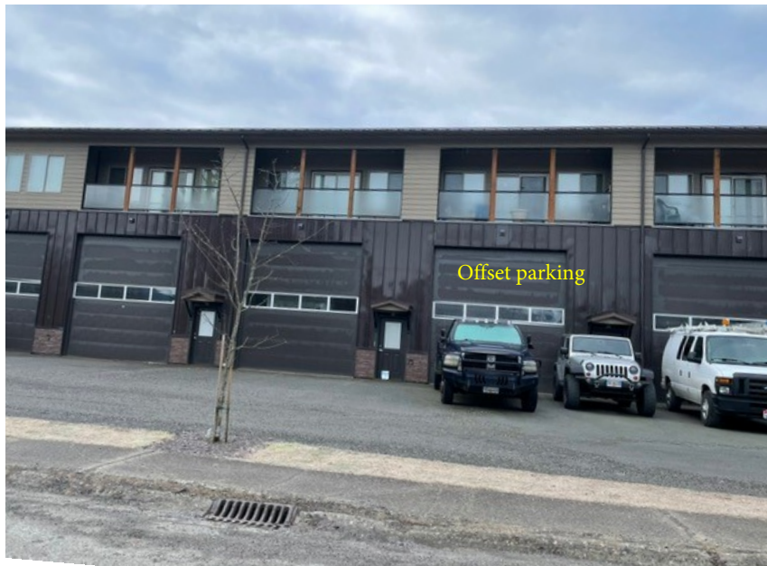
Attachment F - Site Photos
