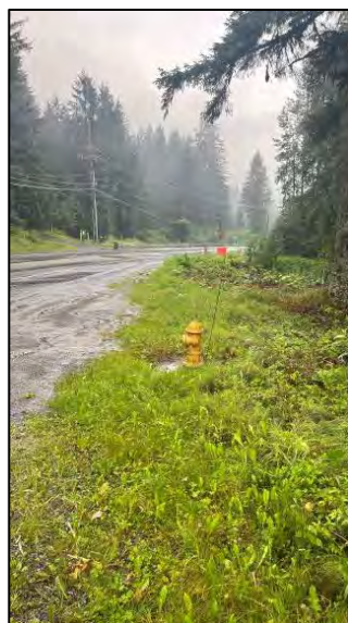
Men. Loop Entrance Looking North
