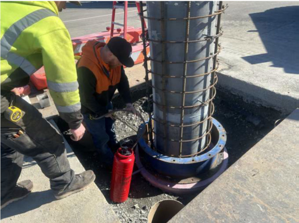
PHOTO 03: Form Base Set in Position at LP-5
