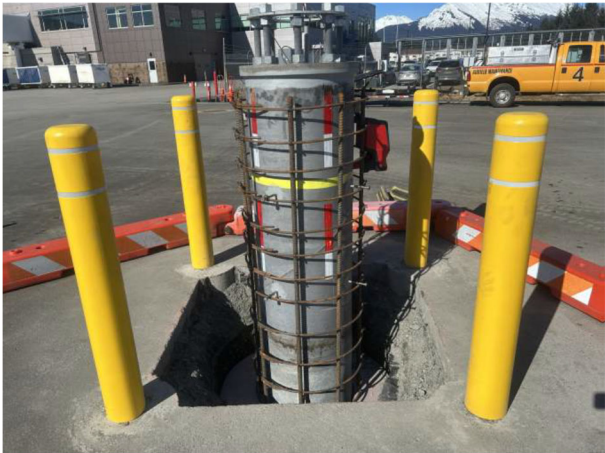
PHOTO 02: Typical Reinforcing Installed Around the Piling
