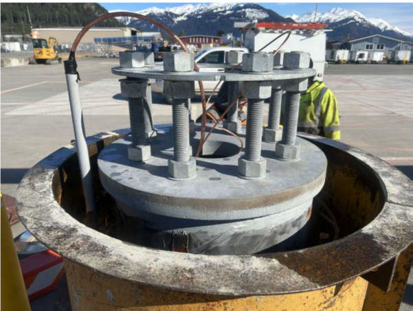
PHOTO 01: Typical Pile Cap Assembly
