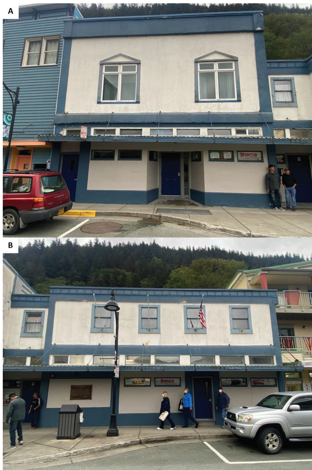
Figure 1. Filipino Community, Inc. Building: left (A) and right (B) sides.
