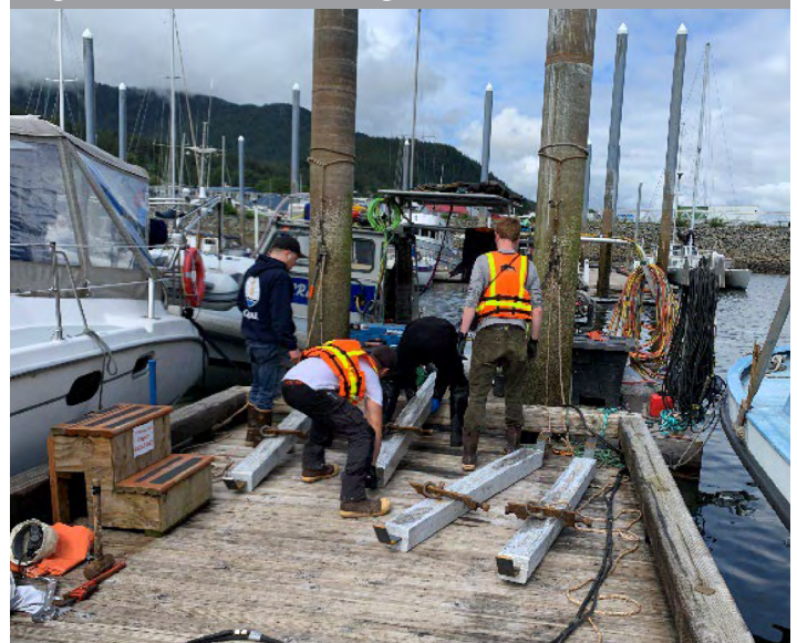
Figure 11: Divers Installing Anodes
