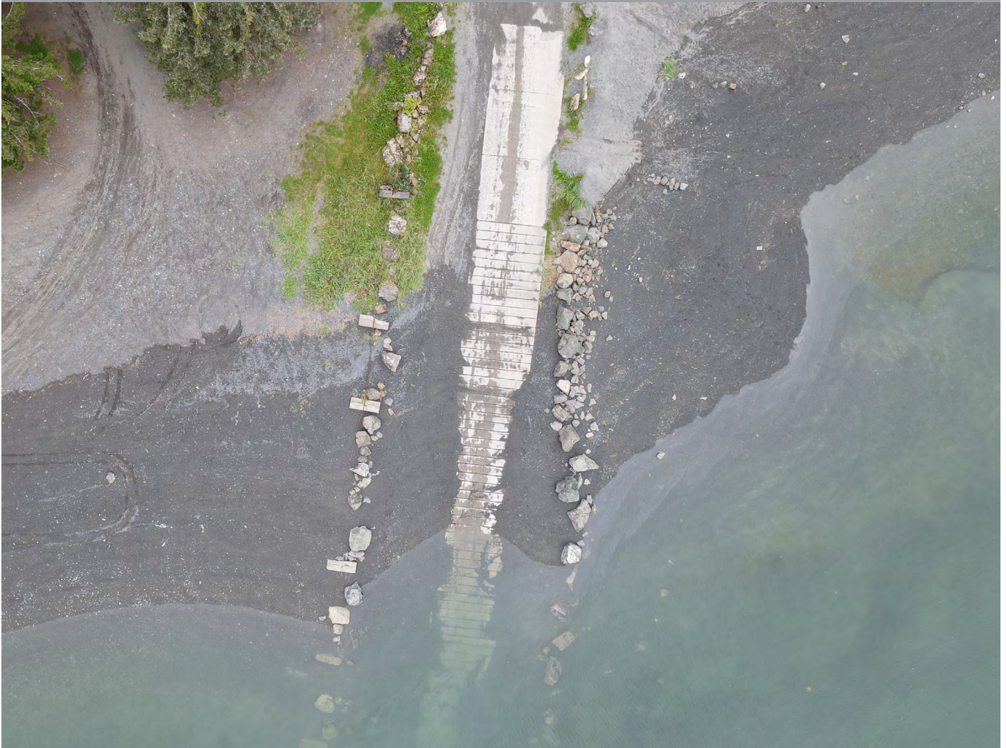
Figure 7: Existing Echo Cove Launch Ramp
