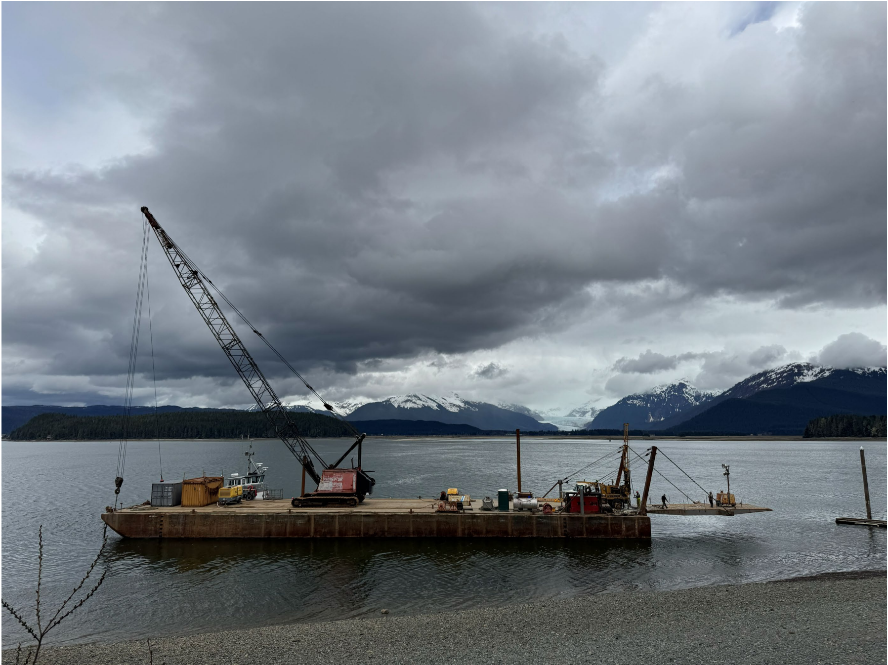
Figure 2- Barge and Drilling Outfit at North Douglas
