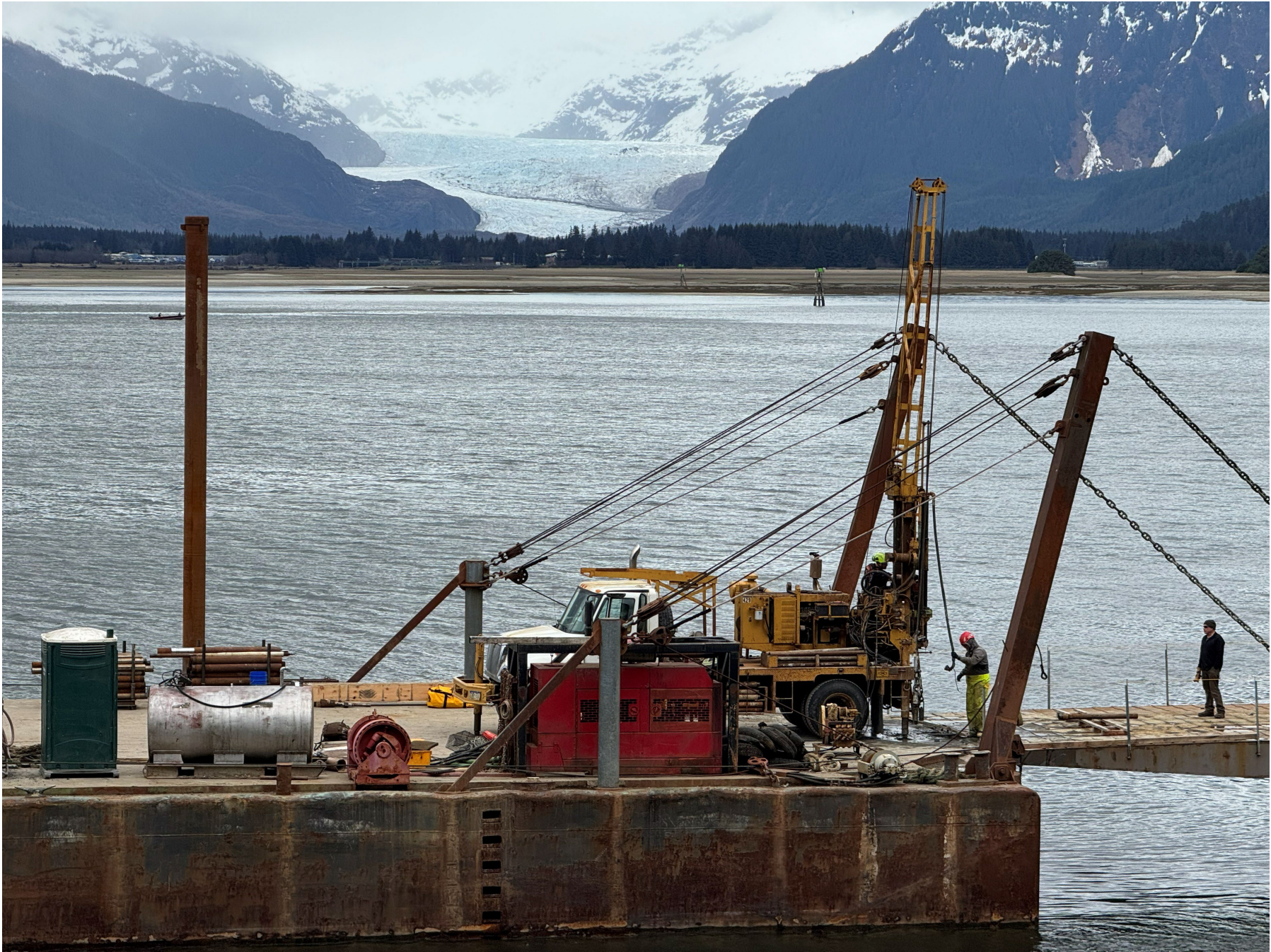
Figure 4 - Drilling Equipment in front of the Glacier
