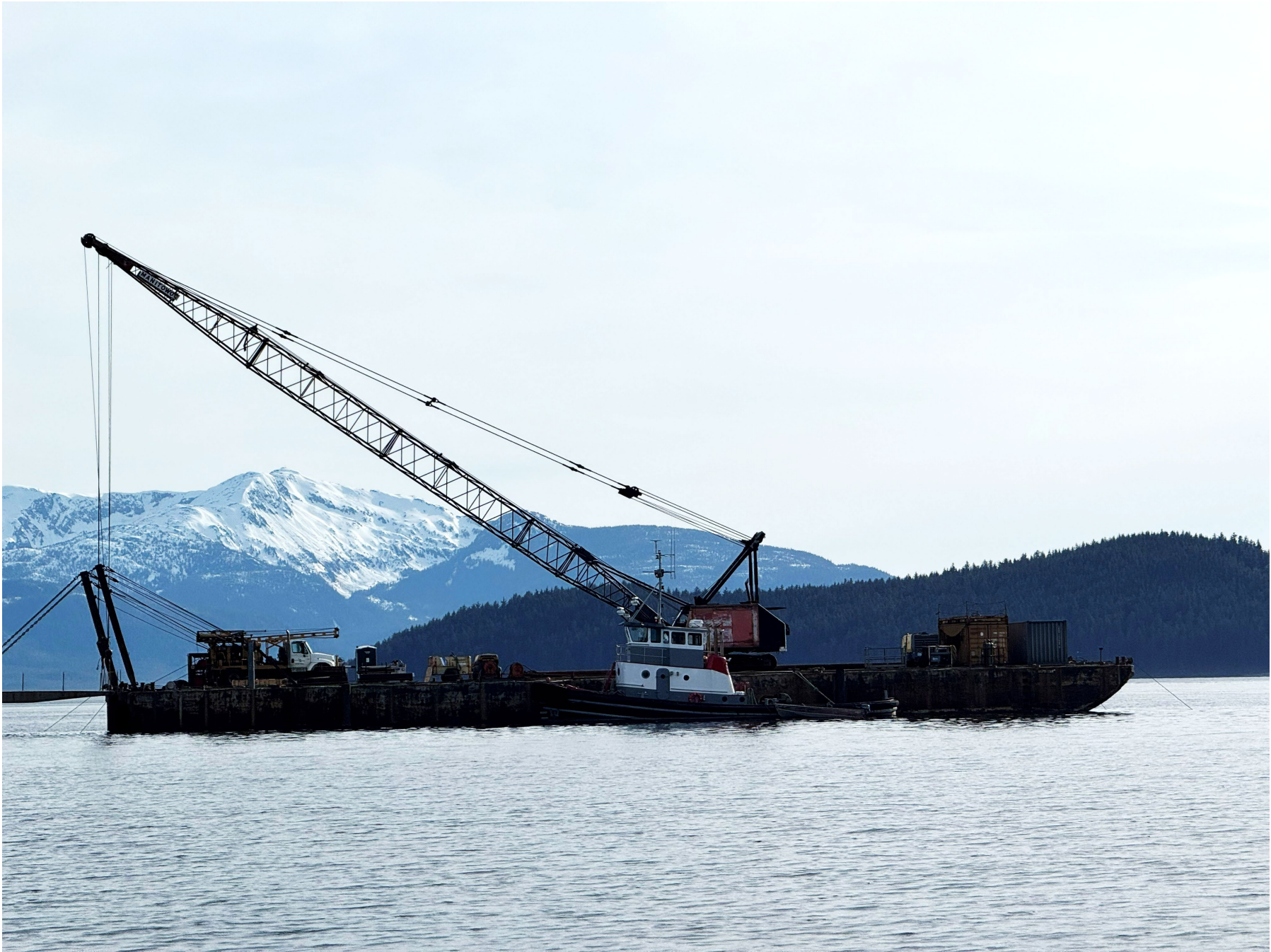
Figure 1- Discovery Drilling and Trucano Construction @ Statter 5/4
