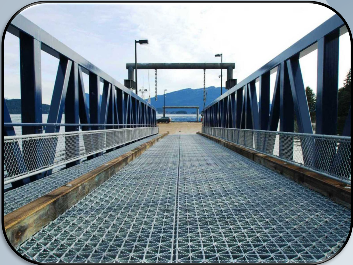
Steel Transfer Bridge Section Auke Bay Loading Facility – Juneau, AK
