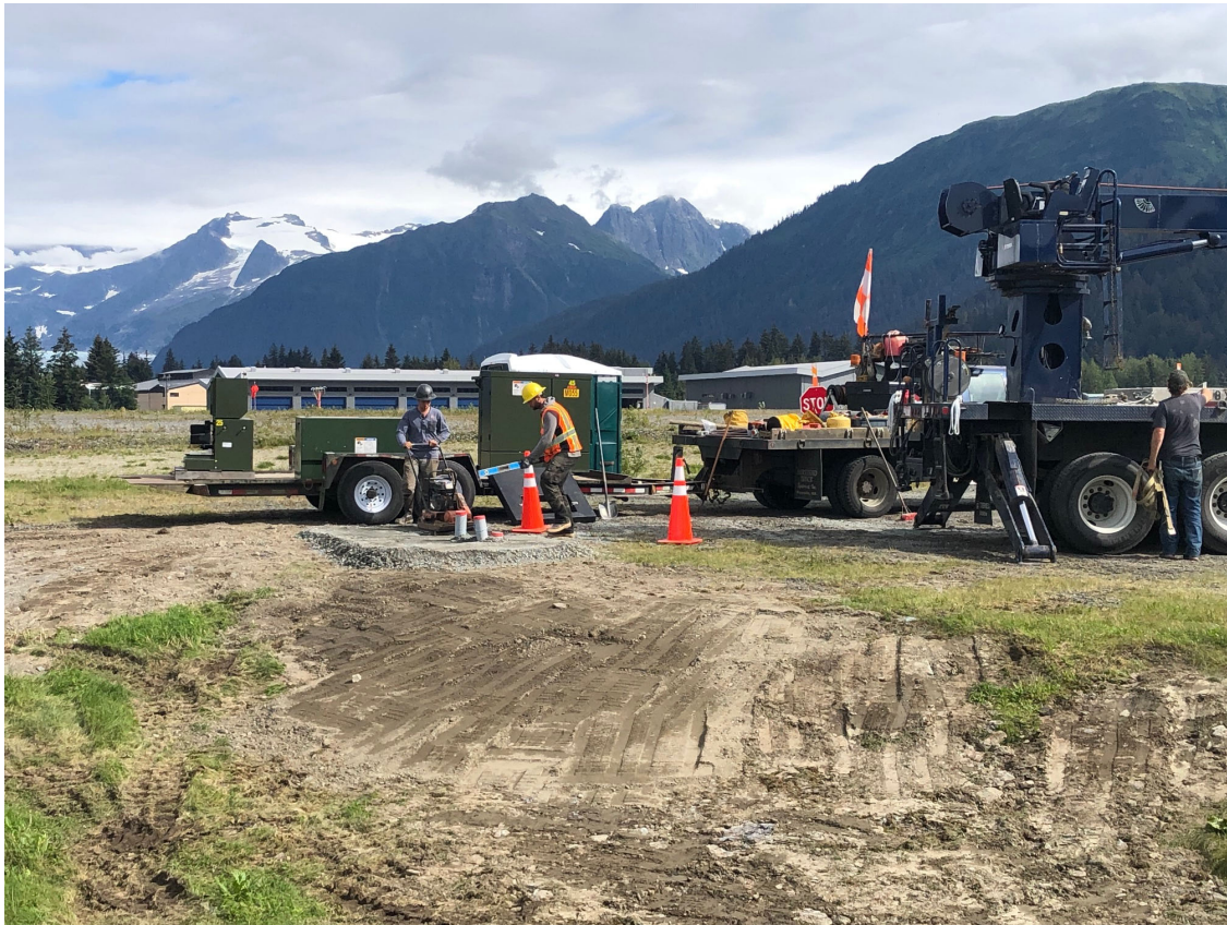
Photo 01: AEL&P preparing the transformer pad near the west end of the float pond.
