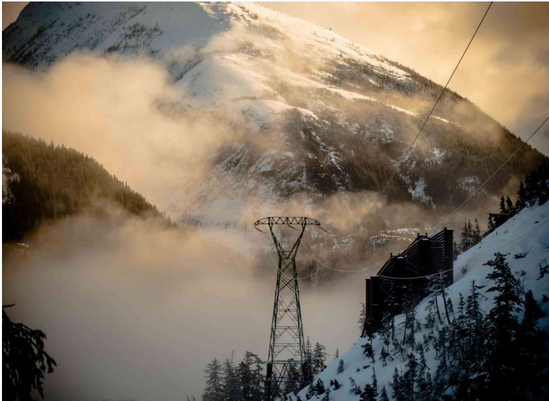
A tower and avalanche diversion wall on the Snettisham transmission line. (Photo courtesy of Mike Janes/AEL&P)
