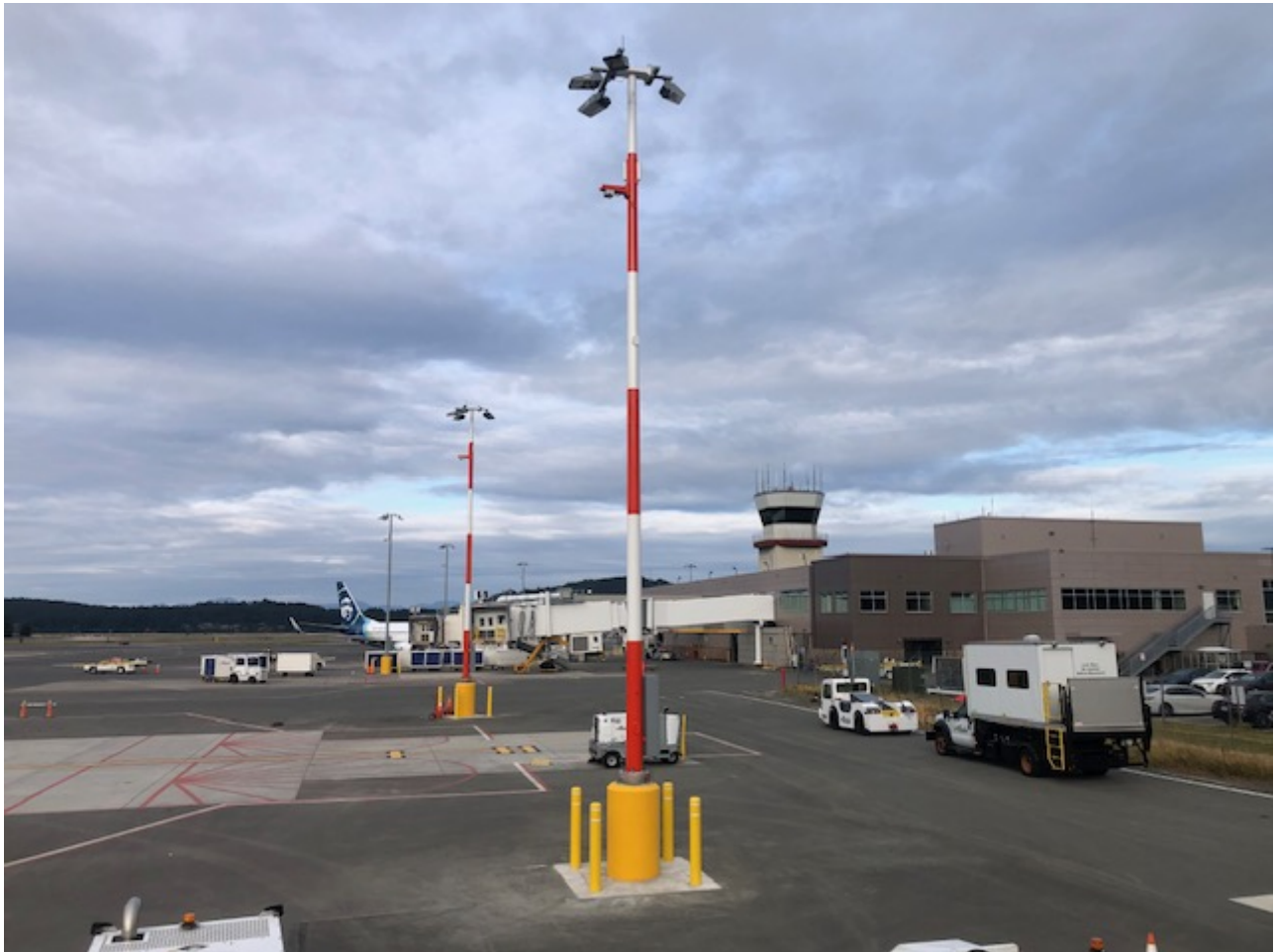
Revised light pole installations – looking west.
