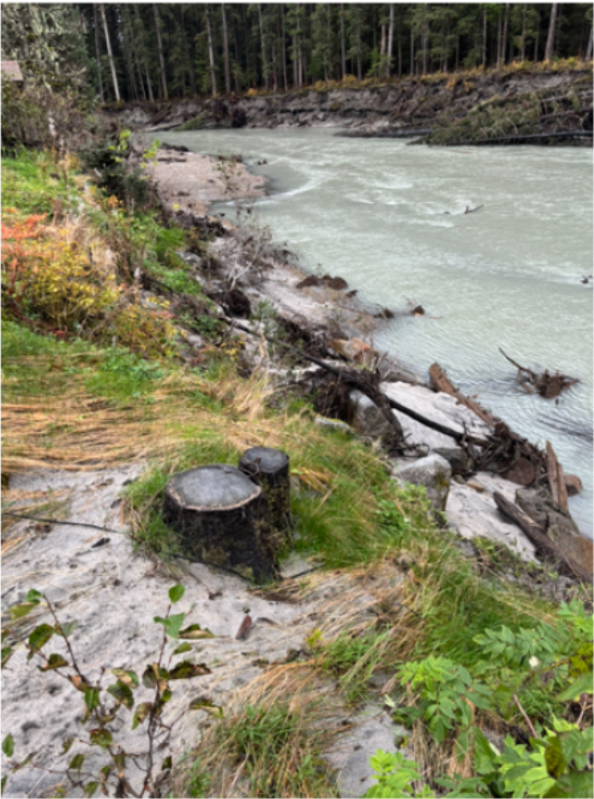
Remaining Bank armoring 3499,3495 Meander Way
