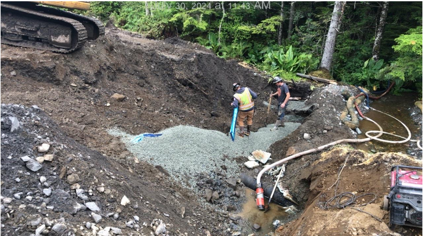
D-1 bedding installed around the water service to 16216 Glacier Hwy.
