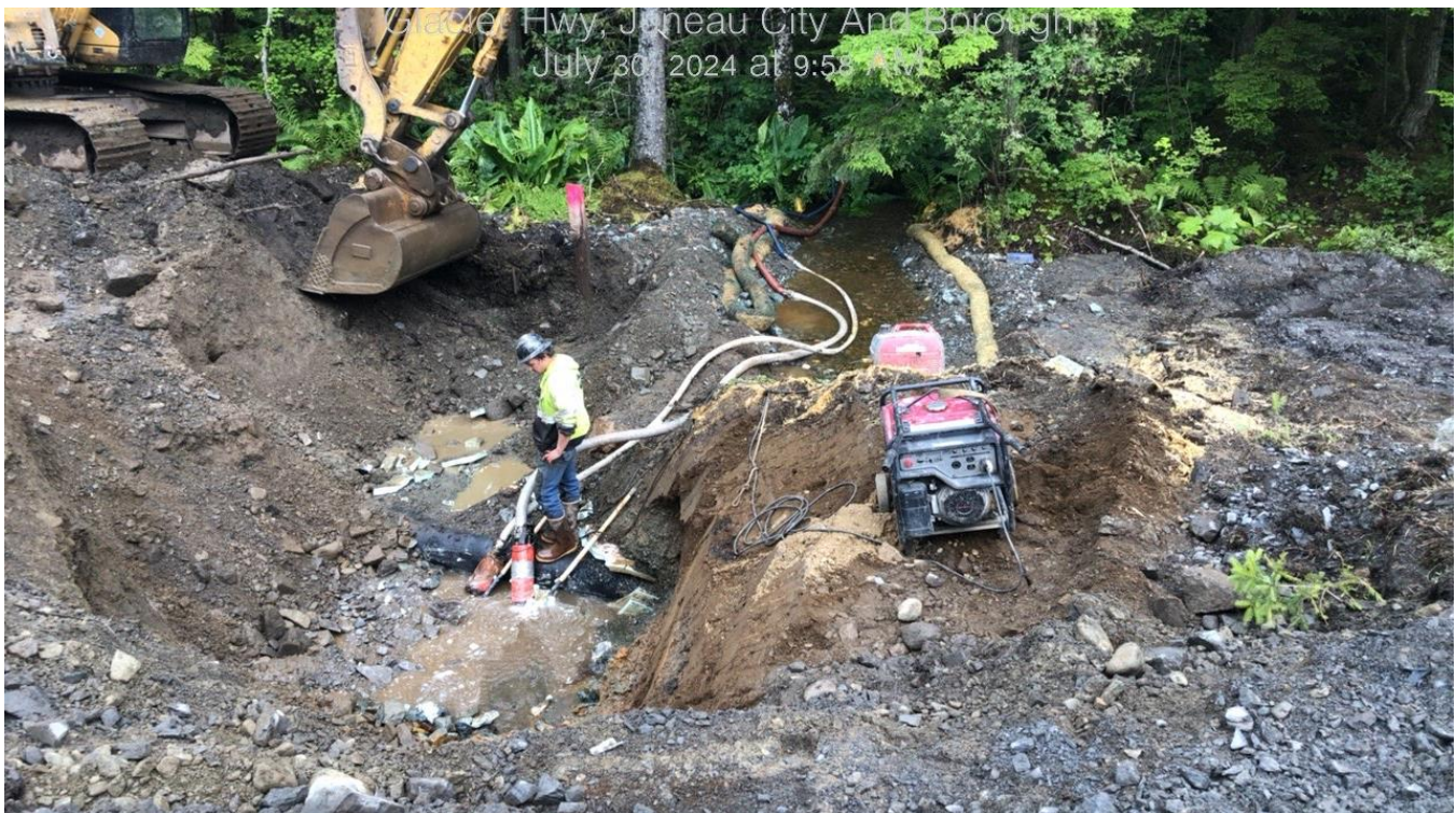
North40 preparing to install the 2-inch water service for 16216 Glacier Hwy.
